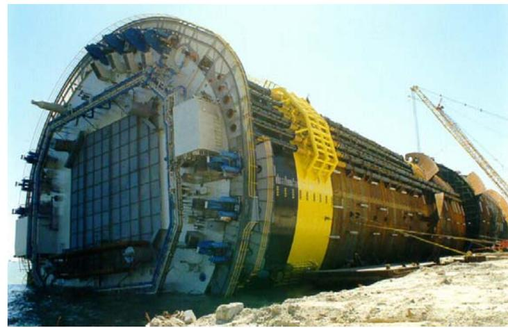
Figure 1 Genesis spar platform under construction showing some of the exterior appurtenances.
